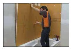
or horizontally on framing with appropriate screws (e.g., coarse thread wood screw for wood studs and self-tapping for metal studs) and corresponding KERDI-BOARD-ZT washers. Minimum board thickness = 1/2" (12.5 mm) for studs spaced at 16" (40.6 cm) o.c.; 3/4" (19 mm) for studs spaced at 24" (61.0 cm) o.c. Screws must reach a depth of at least 3/4" (20 mm) in wood studs and at least 3/8" (10 mm) in metal studs.
