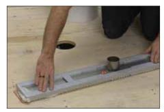
Apply Schluter SET™, ALL-SET™, FAST-SET™, or unmodified thin-set mortar to the top of the channel support with a notched trowel and press the channel support firmly onto the underside of the channel body. Attach the mechanical coupling to the drain outlet and the cut section of the pipe per the coupling manufacturer's instructions.
