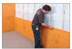
1 KERDI-BOARD can be mounted vertically or horizontally on framing with appropriate screws (i.e., coarse thread wood screw for wood studs and self-tapping for metal studs) and corresponding KERDI-BOARD-ZT washers. Minimum board thickness = 1/2" (12.5 mm) for studs spaced at 16" (40.6 cm) o.c.; 3/4" (19 mm) for studs spaced at 24" (61.0 cm) o.c. Screws must reach a depth of at least 3/4" (20 mm) in wood studs and at least 3/8" (10 mm) in metal studs.
