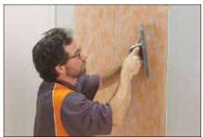
Apply Schluter SET™, ALL-SET™, FAST-SET™, or unmodified thin-set mortar using a 1/4" x 3/16" (6 mm x 5 mm) V-notched trowel or the KERDI-TROWEL. Embed KERDI or KERDI-DS in the mortar and work the membrane onto the entire surface to ensure full coverage and remove air pockets.
