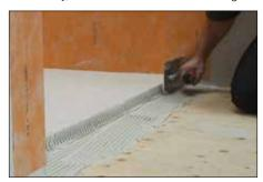
Apply Schluter SET™, ALL-SET™, FAST-SET™, or unmodified thin-set mortar to the floor and to the edge of the shower base and walls using a 1/4" x 3/8" (6 mm x 10 mm) square- or U-notched trowel.
