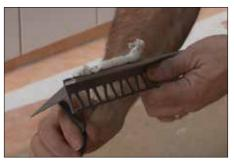
Place the tapered profile into the support section and apply Schluter SET™, ALL-SET™, FAST-SET™, or unmodified thin-set mortar to the fleece on the back side of the profile.
