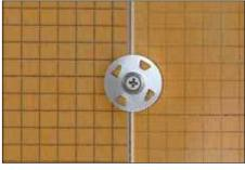
2 Abut panels over the center of the studs or other solid backing. Screws may be placed between adjacent panels such that the washers fasten both panel edges. The maximum allowable on-center fastener spacing is 12" (30 cm) for walls and 6" (15 cm) for ceilings.
