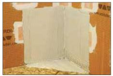
Apply Schluter SET<sup>™</sup>, ALL-SET<sup>™</sup>, FAST-SET<sup>™</sup>, or unmodified thin-set mortar to the floor and walls using a 1/4" x 3/8" (6 mm x 10 mm) square- or U-notched trowel.
