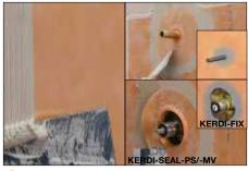
3 Seams in the membrane are constructed by overlapping the edges by 2" (50 mm) or by abutting adjacent sheets and installing KERDI-BAND, centered over the joint. Any protrusions through the membrane (e.g., mixing valve, shower head, etc.) must be sealed with KERDI-SEAL-PS/-MV, KERDI-FIX, or other suitable sealant.
