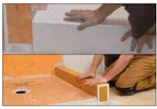
Press the curb or ramp firmly into place. Check the underside of the curb or ramp to ensure that full coverage and support is achieved. Note: When setting tile on the curb, the surface must be sloped towards the shower drain.
