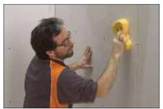
1 Clean any dust or other debris from the surface of the solid backing. Dampen particularly dry and porous substrates in order to help prevent premature drying or skinning of the thin-set mortar.
