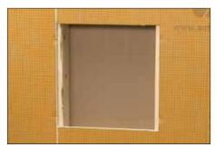
Determine desired location and trace around the outside of the KERDI-BOARD-SN flange, making sure the lines are level and plumb. Cut and remove the KERDI-BOARD such that the niche will be supported on both sides by the studs or other wall framing.
