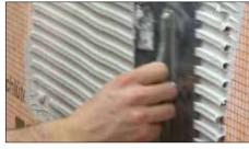
Once all seams and corners have been completely sealed, the assembly is waterproofed and ready to be tiled. Apply a uniform layer of Schluter SET™, Schluter ALL-SET™, Schluter FAST-SET™, or unmodified thin-set mortar and comb using a trowel that is appropriate for the size of the tile. Be sure the trowel groves in the thin-set are all going the same direction, as shown in the photo above.
