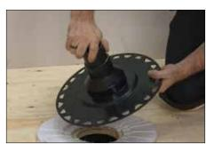
Begin by dry-fitting the components. Measure and cut a section of pipe to connect KERDI-DRAIN to the odor trap using the detachable center section of the tray or foam spacers included with the drain as a spacer. Prepare the odor trap, pipe, and KERDI-DRAIN with cleaner, primer and ABS or PVC cement per the solvent cement manufacturer's instructions and connect.
