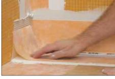
3 The KERDI collar on KERDI-LINE is integrated with the adjoining waterproofing assembly using Schluter SET™, ALL-SET™, FAST-SET™, or unmodified thin-set mortar. The KERDI collar must be cut and folded where the KERDI-LINE is installed adjacent to walls.
