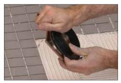
Place the height adjustment collar inside the lateral adjustment ring and snap the grate into place. **Note:** For the 6" (150 mm) grates, the height adjustment collar is integrated with the grate. For the residential adaptor kit, there is no lateral adjustment ring.
