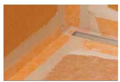
Seams in the membrane are constructed by overlapping the edges by 2" (50 mm) with Schluter SET™, ALL-SET™, FAST-SET™, or unmodified thin-set mortar or by abutting adjacent sheets and installing KERDI-BAND with unmodified thin-set mortar, centered over the joint.
