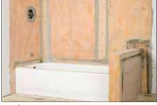
Once the entire membrane, including seams, corners, and knee walls have been completely bonded and, therefore, waterproofed, the assembly is ready to be tiled. For tile installation instructions, see page 30.
