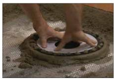
Place a ring of loose mortar up to the inlet hole in the floor and firmly press the drain into the mortar and level. The bonding flange must be fully supported to prevent damage to the tile assembly (e.g., cracked grout around drain). When installing KERDI-DRAIN over wood substrates, the minimum thickness of mortar required at the perimeter of the bonding flange is 1" (25 mm).
