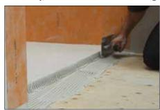
Apply Schluter SET<sup>™</sup>, ALL-SET<sup>™</sup>, FAST-SET<sup>™</sup>, or unmodified thin-set mortar to the floor and to the edge of the shower base and walls using a 1/4" x 3/8" (6 mm x 10 mm) square- or U-notched trowel.
