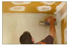
Apply Schluter SET™, ALL-SET™, FAST-SET™, or unmodified thin-set mortar to the shower base with a 1/4" x 3/16" (6 mm x 5 mm) V-notched trowel or the KERDI-TROWEL. The thin-set mortar must be mixed to a fairly fluid consistency, but still able to hold a notch.
