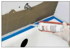
Place painter's tape to protect the tub deck. Apply Schluter SET™, ALL-SET™, FAST-SET™, or unmodified thin-set mortar to the solid backing using a 1/4" x 3/16" (6 mm x 5 mm) V-notched trowel or the KERDI-TROWEL. Completely fill the 1/4" (6 mm)-wide gap between the solid backing and tub with KERDI-FIX or other suitable sealant. Note: When the solid backing is installed above the tub flange, apply KERDI-FIX to the tub flange and spread using a small notched trowel.
