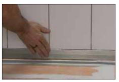
Apply Schluter SET™, ALL-SET™, FAST-SET™, or unmodified thin-set mortar to the fleece on the back side of the profile. Press the profile into place and align it flush with the wall tile. Immediately clean away any excess setting material.
