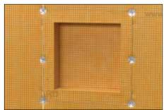
Insert the niche and fasten to the studs using wood or metal screws and KERDI-BOARD-ZT washers, placing the fasteners along the seam between the KERDI-BOARD and the niche. Fasten all corners and limit fastener spacing to 12" (30 cm) o.c.
