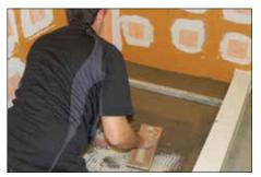
Fill the remainder of the shower base with mortar and slope the mortar bed at 1/4" (6 mm) per 12" (305 mm) using the bonding flange and a perimeter screed as guides.
