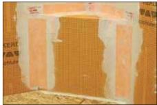
Install KERDI-BAND and KERDI-KERECK and KERDI-KERS-B (for triangular bench) to cover all seams and corners, ensuring a minimum 2" (50 mm) overlap, and work the membrane into the mortar to achieve full coverage and remove air pockets.
