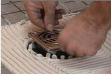
2 Fill the step in the bonding flange with thin-set mortar and back-butter the underside of the grate to ensure full support. Place the assembly into the mortar and install the surrounding tiles, ensuring full coverage.
