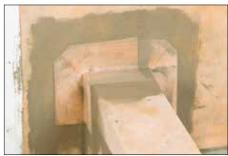
Seal connections to knee walls using KERDI-KERECK-F preformed corners and Schluter SET™, ALL-SET™, FAST-SET™, or unmodified thin-set mortar.
