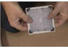
2 Apply tile to the top of the covering support using Schluter SET™, ALL-SET™, FAST-SET™, or unmodified thin-set mortar. The tile may overhang the covering support provided that a drainage opening of at least 3/16" (5 mm) is provided.
