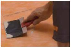
Embed KERDI or KERDI-DS in the bond coat and work the membrane onto the entire surface to ensure full coverage and remove air pockets. The membrane is carried to the stainless steel bonding flange and to the edges of the shower base.
