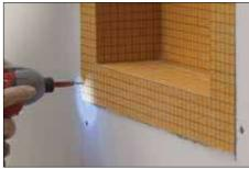
Insert the niche and fasten to the studs using wood or metal screws, placing the fasteners approximately 1/4" (6 mm) from the edges of the niche. Fasten all corners and limit fastener spacing to 12" (30 cm) o.c.
