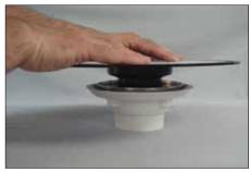
Slide the adaptor flange into the adaptor ring and ensure full support under the adaptor flange with mortar. The mortar bed is then placed according to the instructions on page 23.
