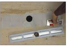
Apply Schluter SET<sup>™</sup>, ALL-SET<sup>™</sup>, FAST-SET<sup>™</sup>, or unmodified thin-set mortar to the substrate where the drain is to be placed with a notched trowel. Prepare the cut section of pipe and odor trap with cleaner, primer and ABS or PVC cement per the solvent cement manufacturer's instructions.
