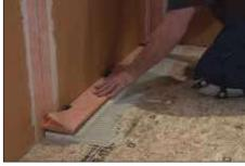
Apply Schluter SET™, ALL-SET™, FAST-SET™, or unmodified thin-set mortar to the top of the channel support and press the channel body firmly into the mortar, ensuring full support of the bonding flange. Check to make sure the KERDI-LINE is level.
