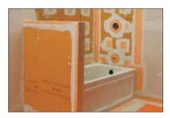
8 Once all seams, corners, and knee walls have been completely sealed, the assembly is waterproofed and ready to be tiled.
