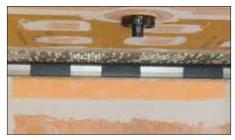
2 Insert the tile spacers into the channel body. Install the surrounding tile on the adjoining walls and shower base up to the spacers using Schluter SET", ALL-SET", FAST-SET", or unmodified thin-set mortar, ensuring full coverage. Remove all excess setting material.
