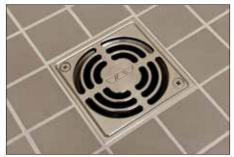
Position the grate to match the joint pattern of the tile covering and press flush with the tile surface. Remove all excess setting material immediately. Note: Protect the visible surface of the grate from contact with setting and grouting materials. In particular, anodized aluminum is sensitive to alkaline materials.
