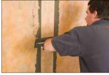
Seams in the membrane are constructed by overlapping the edges of KERDI by 2" (50 mm) or by abutting adjacent sheets of KERDI and installing KERDI-BAND, centered over the joint.
