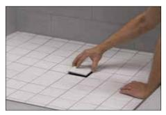
3 After the tile is set and grouted, remove the tile spacer and insert the tiled covering support into the lateral adjustment ring.
