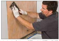
4 Apply Schluter SET™, ALL-SET™, FAST-SET™, or unmodified thin-set mortar to the solid backing and previously applied KERDI-BAND. Embed the KERDI in the thin-set mortar and work the membrane onto the entire surface to ensure full coverage and remove air pockets.
