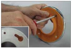
1 Remove the clamping ring from the installed drain and save the bolts. Align the bolt pattern of the clamping ring with the adaptor ring and punch the matching inserts through the adaptor ring.
