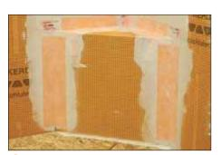
Install KERDI-BAND and KERDI-KERECK and KERDI-KERS-B (for triangular bench) to cover all seams and corners, ensuring a minimum 2" (50 mm) overlap, and work the membrane into the mortar to achieve full coverage and remove air pockets.
