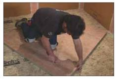
Any leveling of the floor must be done prior to the installation of the shower tray. If necessary, cut the tray to size prior to application. The shower base can also be extended beyond the tray using dry-pack mortar, which is in turn covered with the KERDI membrane.
