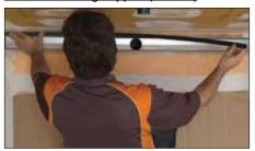
1 Peel the protective foil off the cover strip and adhere the strip to the bonding flange adjacent to the wall(s). Position the strip along the edge of the channel. The cover strip hides and protects the KERDI surface under the tile installed in step 3.
