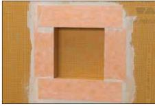
Seal the seams between the niche and walls using KERDI-BAND with Schluter SET™, ALL-SET™, FAST-SET™, or unmodified thin-set mortar ensuring a 2" (50 mm) overlap in all directions.
