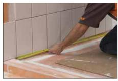
1 Measure the height of the area to be covered at the lowest point. Next, measure the length of the area and mark the profile where it is to be cut at both ends. Remove the protective foil and cut the tapered profile and support section to length
