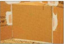
Press the bench firmly into place and check the underside and backsides to ensure that full coverage and support are achieved. Verify that the slope on the surface of the bench is directed toward the shower base.
