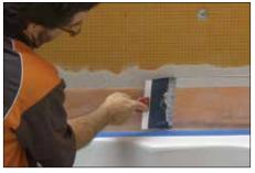
Apply KERDI-BAND waterproofing strips. Solidly embed the membrane in the mortar and KERDI-FIX to ensure full coverage and remove air pockets.
