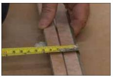
Connect the two components of SHOWERPROFILE-R to achieve the desired height. Small pieces of tape can be used to help maintain the position of the components during installation.
