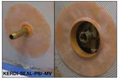
6 Any protrusions through the panel (e.g., mixing valve, shower head, etc.) must be sealed with KERDI-SEAL-PS/-MV, KERDI-FIX, or other suitable sealant.
