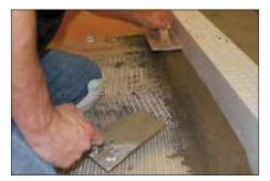
Place a mortar screed opposite the installed KERDI-LINE channel body.
