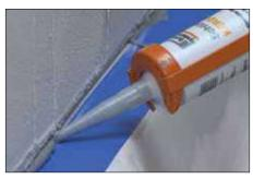
Place painter's tape to protect the tub deck. Apply Schluter SET™, ALL-SET™, FAST-SET™, or unmodified thin-set mortar to the KERDI-BOARD using a 1/4" x 3/16" (6 mm x 5 mm) V-notched trowel or the KERDI-TROWEL. Completely fill the 1/4" (6 mm)-wide gap between the KERDI-BOARD and tub with KERDI-FIX or other suitable sealant.
