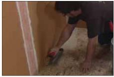
Apply Schluter SET<sup>™</sup>, ALL-SET<sup>™</sup>, FAST-SET<sup>™</sup>, or unmodified thin-set mortar to the substrate where the drain is to be placed with a notched trowel and solidly embed the channel support in the mortar.
