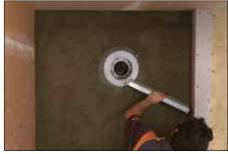
The screed is then placed flush with the top of the bonding flange of the KERDI-DRAIN. Slope the mortar bed at 1/4" (6 mm) per 12" (305 mm) using the bonding flange and a perimeter screed as guides.
