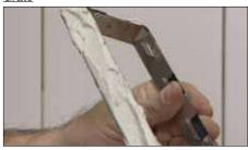
Apply Schluter SET™, ALL-SET™, FAST-SET™, or unmodified thin-set mortar to the underside of the grate frame and place it in the channel body ensuring full coverage and support of the frame. Insert the foam spacers in the grate frame to reinforce it during the remainder of the installation.
