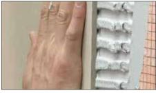
Solidly embed the tiles in the setting material, making sure to observe the open time of the bonding mortar. If the mortar skins over prior to tile installation, remove and reapply.
