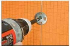
Abut panels over the center of the studs. Screws may be placed between adjacent panels such that the washers fasten both panel edges. The maximum allowable on-center fastener spacing is 12" (30 cm) for walls and 6" (15 cm) for ceilings.
