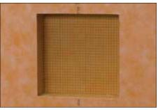
Apply the KERDI membrane over the wall surface as described on page 20. Once the membrane is solidly embedded, cut the membrane to match the niche opening.
