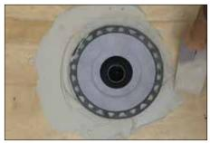
Apply Schluter SET™, ALL-SET™, FAST-SET™, or unmodified thin-set mortar to the substrate and to the top and bottom of the detached center section of the KERDI-SHOWER-T/-TS/-TT tray. Slide the center section into place below the drain to ensure solid and uniform support of the bonding flange.
