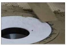
Pack loose mortar under the drain up to the inlet hole to ensure solid and uniform support of the bonding flange and level. The mortar bed is then placed according to the instructions above.
