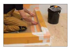
When using KERDI-SHOWER-SC/-SR, repeat the process to install the membrane over the curb or ramp. Seams in the membrane are constructed by overlapping the edges by 2" (50 mm) or by abutting adjacent sheets and installing KERDI-BAND centered over the joint. Install KERDI-KERECK at all inside and outside corners. When using KERDI-BOARD-SC, seal the curb to the base and walls using KERDI-KERECK and KERDI-BAND.
