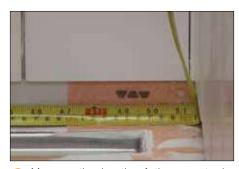
Measure the length of the area to be covered. Remove the protective foil and cut the profile to length.
