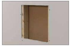
1 Determine desired location and trace around the outside of the KERDI-BOARD-SN flange, making sure the lines are level and plumb. Cut and remove the wallboard such that the niche will be supported on both sides by the studs or other wall framing.
