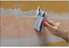
KERDI-BOARD joints, corners, and fastener penetrations are sealed with KERDI-BAND, ensuring a minimum 2" (50 mm) overlap.
