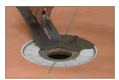
3 Apply Schluter SET™, ALL-SET™, FAST-SET™, or unmodified thin-set mortar to the substrate using a 1/4" x 3/8" (6 mm x 10 mm) square- or U-notched trowel. Place the KERDI-SHOWER-T/-TS/-TT tray and solidly embed in the mortar. Check the underside of the tray to ensure full coverage and support are achieved.
