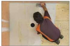
Apply Schluter SET<sup>™</sup>, ALL-SET<sup>™</sup>, FAST-SET<sup>™</sup>, or unmodified thin-set mortar to the substrate using a 1/4" x 3/8" (6 mm x 10 mm) square- or U-notched trowel.
