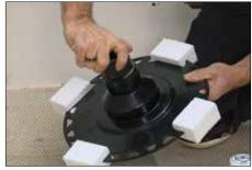
Measure and cut a section of pipe to connect KERDI-DRAIN to the odor trap using the foam spacers included with the drain as a spacer. When installing KERDI-DRAIN over wood substrates, the minimum thickness of mortar required at the perimeter of the bonding flange is 1" (25 mm). Prepare the odor trap, cut section of pipe, and KERDI-DRAIN with cleaner, primer and ABS or PVC cement per the solvent cement manufacturer's instructions and connect.
