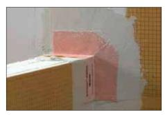
Seal connections to knee walls using KERDI-KERECK-F preformed corners and Schluter SET™, ALL-SET™, FAST-SET™, or unmodified thin-set mortar.
