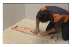
Solidly embed the channel support and KERDI-LINE into the mortar on the floor and connect the cut section of pipe to the odor trap. Check to make sure the KERDI-LINE is level.
