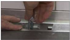
Slide the plastic height adjustment spacers with threaded bolts onto the tabs along the inside of the grate frame to adjust the elevation of the frame. The spacers may be adjusted simply by turning the bolts by hand. The elevation should be set such that the frame will be flush with the surface of the tile covering.
