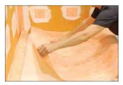
3 As soon as the mortar bed can be walked upon, waterproofing with the KERDI membrane can begin.
