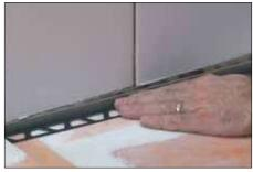
Press the profile into place and align it flush with the wall tile. Immediately clean away any excess setting material. Install adjacent tiles on the shower base.
