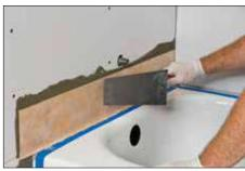
Apply KERDI-BAND waterproofing strips or 5" (125 mm)-wide cut sections of KERDI waterproofing membrane. Solidly embed the membrane in the mortar and KERDI-FIX to ensure full coverage and remove air pockets.
